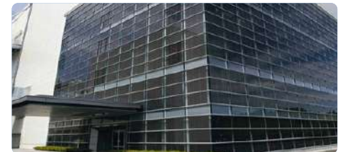
Sharp Kameyama Factory, 112 kWdc
